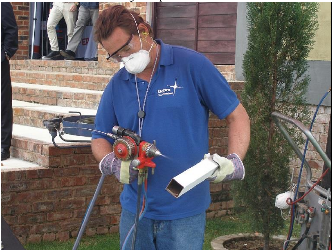
Above: application of the zinc coating through a feeder nozzle
